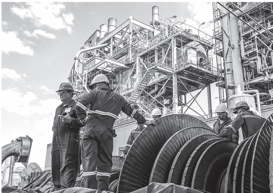
NO TO PRIVATIZATION. Workers of Unión Eléctrica (Cuba's electrical power company) during maintenance work on the thermoelectric power plant in Camagüey, April 2025. The products of the toil and sweat of the working class must not be handed over to the capitalists.
